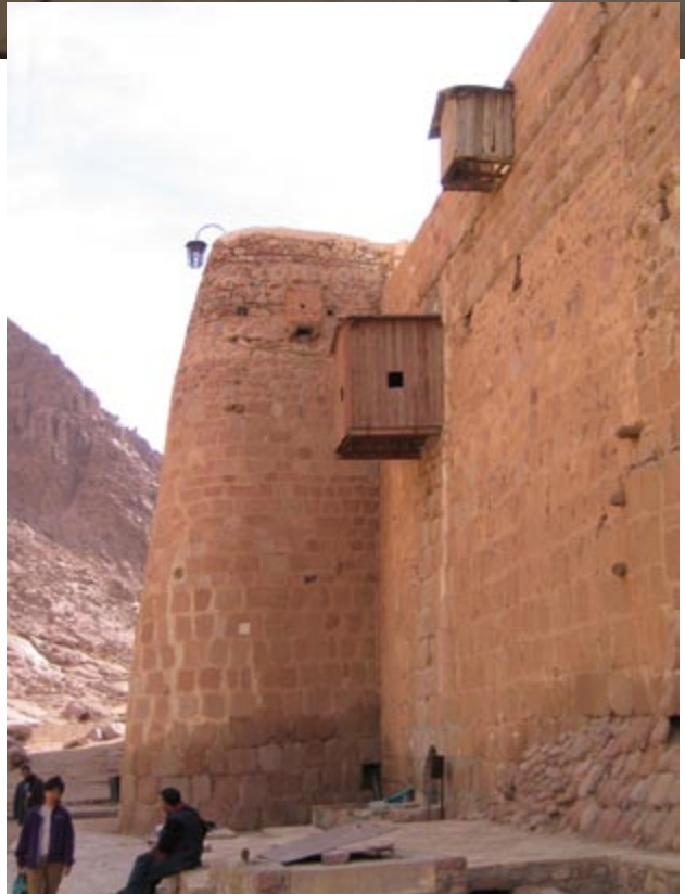
p. 146 - The main door of the structure ... 30 feet above the level of the desert, with no stairs
